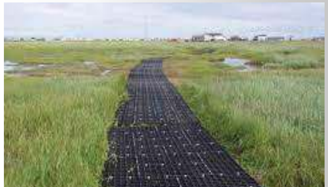
Figure 2 Successful geo-mat installed in rural Alaska
