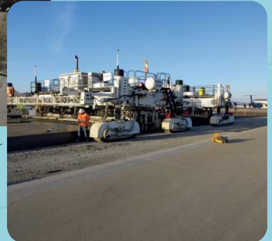
End product of 17 1/2" thick paving
