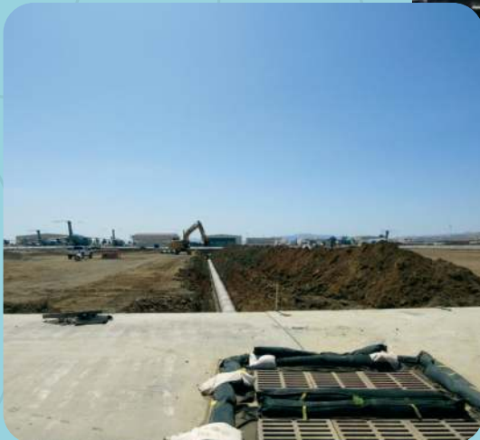
Storm drain installation
